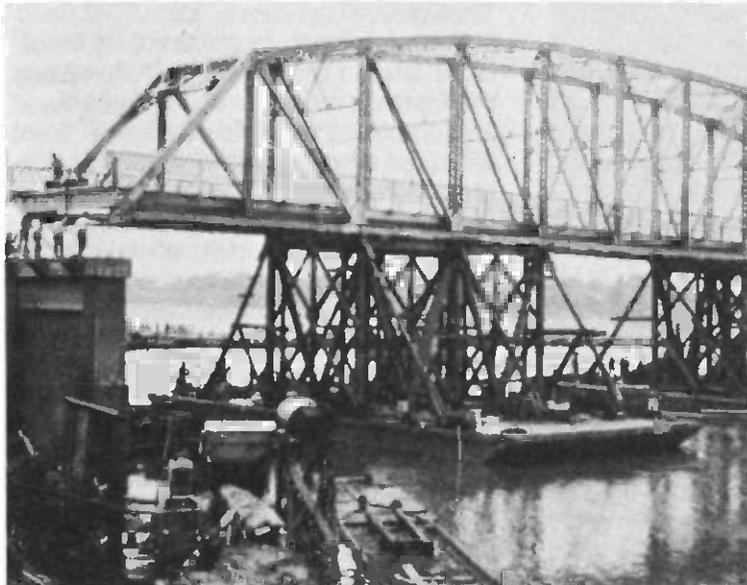
Spans are being lowered onto the piers after being assembled on the river bank and floated to midstream.
