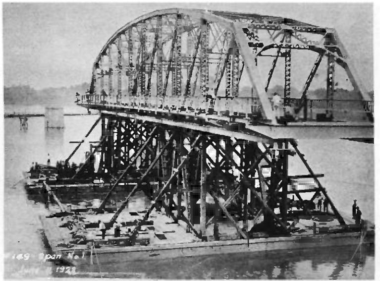
This is the first span of the new bridge that replaced the Pontoon Bridge. After being built on the river bank, the span was floated into place on barges, the water was pumped into the barge and the span would rest on its piers. The barges would move down stream and the water removed. Then they returned to shore for the next span. (June 11, 1928)
